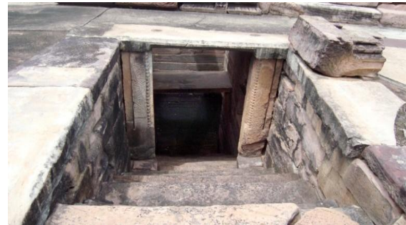
The figure is showing the steps going downwards to the water tank
